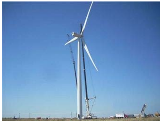
The Alstom wind turbine at Reese Technology Center at the former Reese Air Force Base in Lubbock, Texas, is 110 meters tall from the tip of its outstretched blade to the ground. The turbine, which has been operating since Nov, 2010, generates 1.67 megawatts of power. It is used for research in the Texas Tech University wind science and engineering program and for training in South Plains College's wind technician program. (Courtesy photo)
